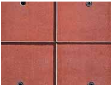
All kinds of colours can be obtained by using pigments and specific fine sands (filler fraction).
