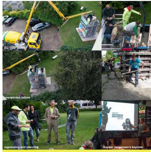
A true truckmixer arrived on the scene for the 'tail one'. Unexpectedly the mould collapsed just before being totally filled. Disappointing indeed! However, no desparation. Plan B was developed, Kasper Jørgensen - GXN - lectured and the last batch of 1:5's was filled.
