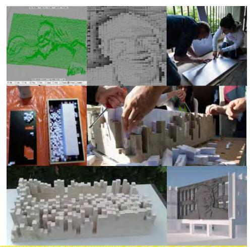
Two approaches combining 'state-of-the-art' digital technology ideas with concrete. A static interpretation of a pixelated media facade. And a seemingly straight-forward sculptural system for which it appeared to be a challenge to built smooth and precise formwork.
